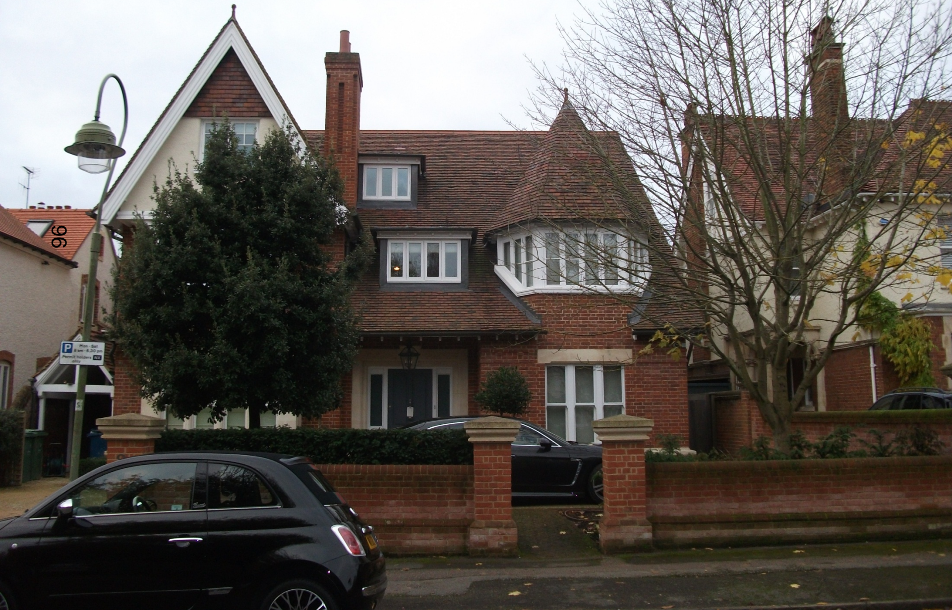
8A Charlbury Road , view of front dormer windows in with the roof
